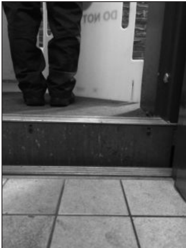
Figure 12: Elevator Car Not Levelling with the Floor
